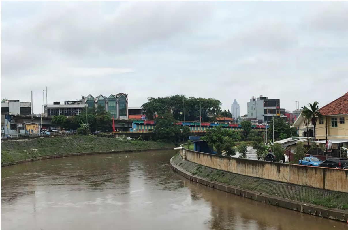
Figure 6. Concrete embankments and walls line the Ciliwung in an effort to protect residential areas from flooding during high water levels (Credit: the authors).
