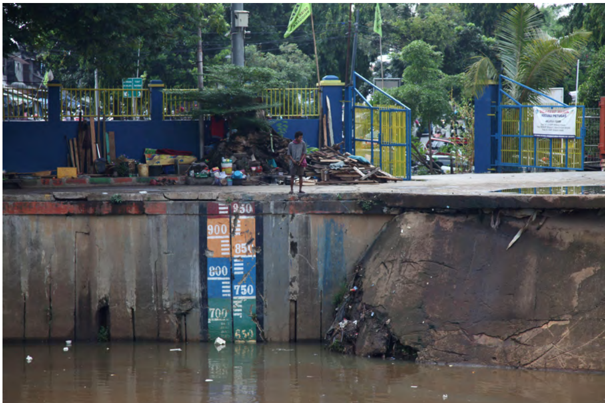
Figure 2. River level measure near the Manggarai floodgate, Jakarta, indicates water height (Pacific Press Media Production Corp./Alamy Stock Photo)
